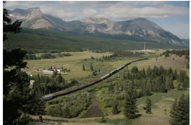
A major freight mainline runs through the region linking British Columbia and Port Metro Vancouver to a major freight handling facility in Lethbridge.
